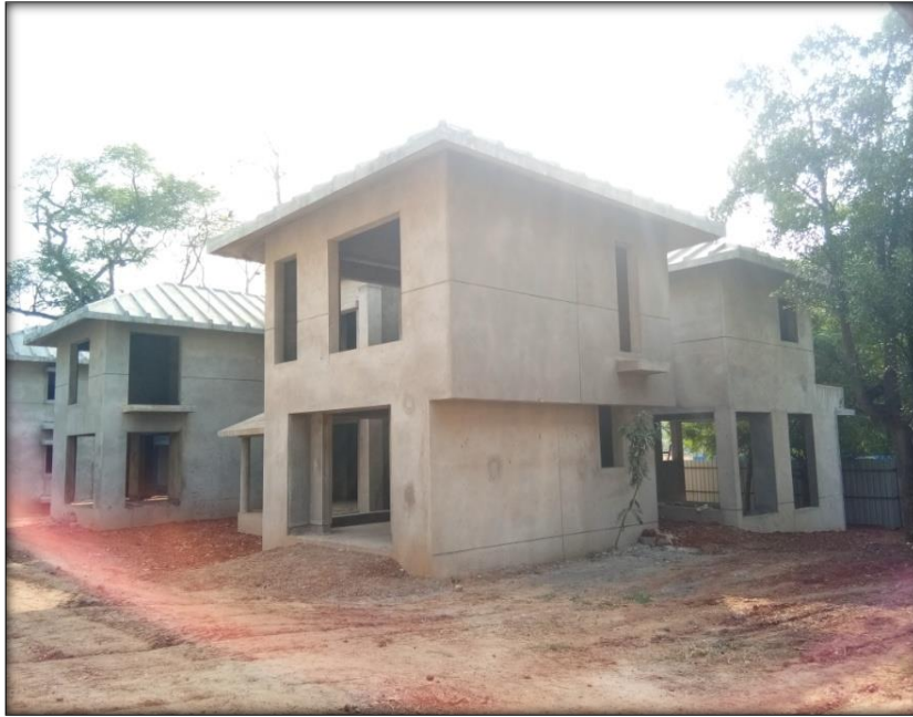
ROOF SLAB WATERPROOFING WORK IN PROGRESS
