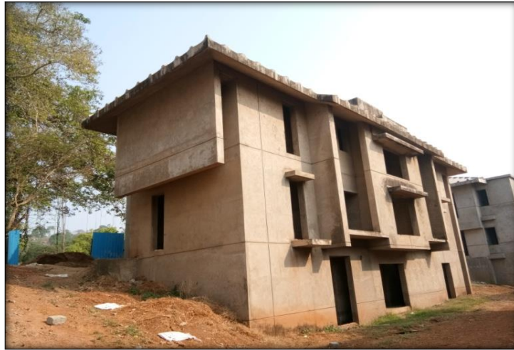
EXTERNAL PLASTER COMPLETE
