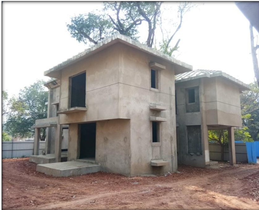
EXTERNAL PLASTER & ROOF WATERPROOFING WORK COMPLETE
