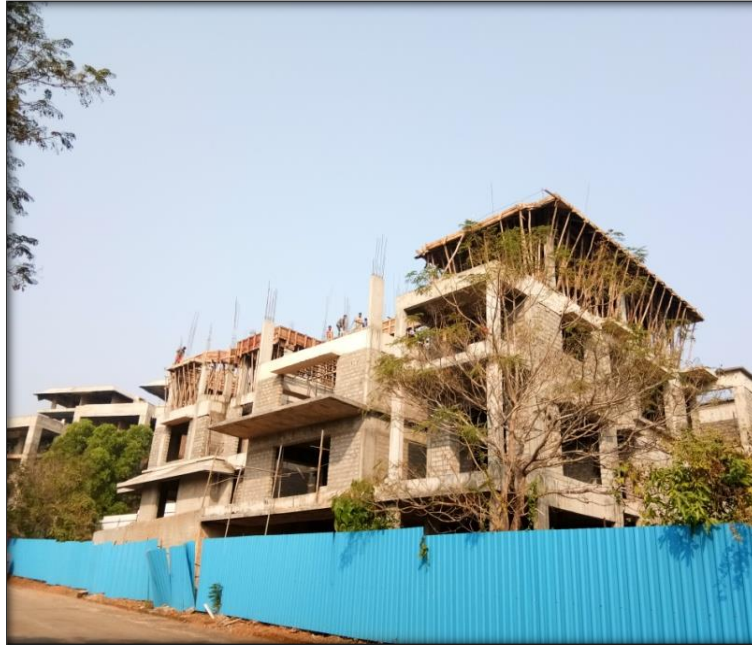
ROOF SLAB WORK & GR. FLOOR MASONRY WORK IN
